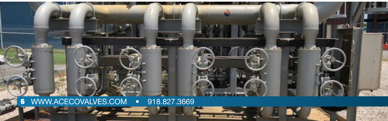
Model BV2 Double Ball Comparison to Conventional Flanged 8" 6000 PSI BV2 vs. 8FP CL 2500
